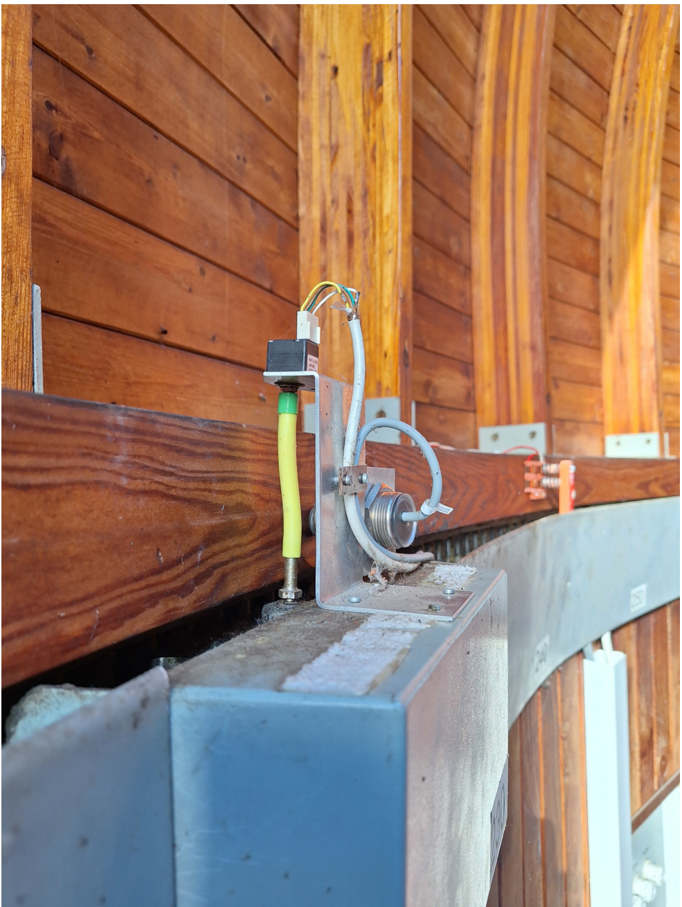
Radio controled slit opening by 12V garage door motor, powered by 12V 15Ah Pb gel accumulator, charged to 13,2V by 2A power source via 3D printed contactor and quadrature encoder with induction sensor for sensing dome position with Shelyak Dome Tracker
