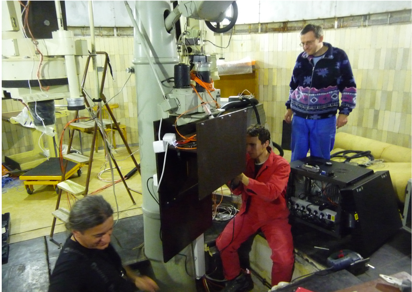
Peter Habaj, Matúš Kozák, Jaro Ambróz installing a box with the CoMP-S electronics
